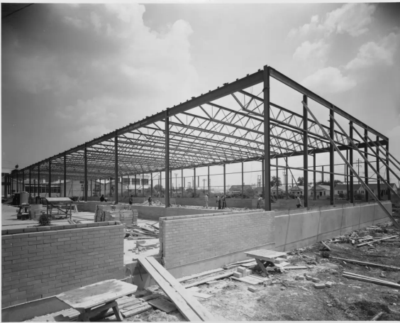
Representative steel construction image
